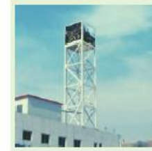
Roof Top Modernization
