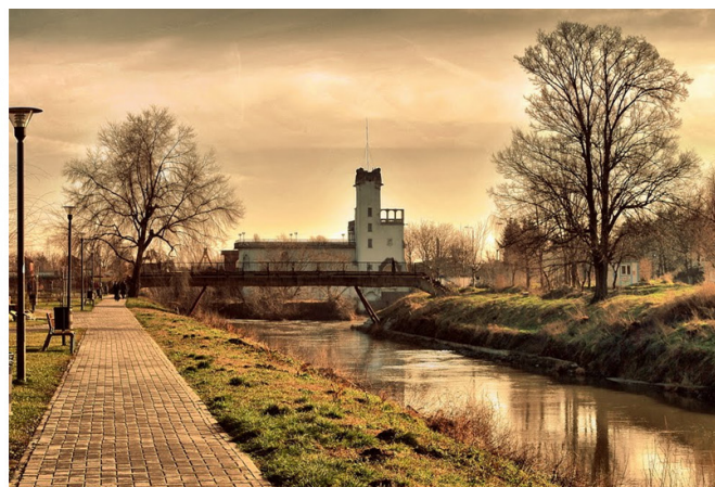
Figure 2. The old power plant (located on the Bega River)
